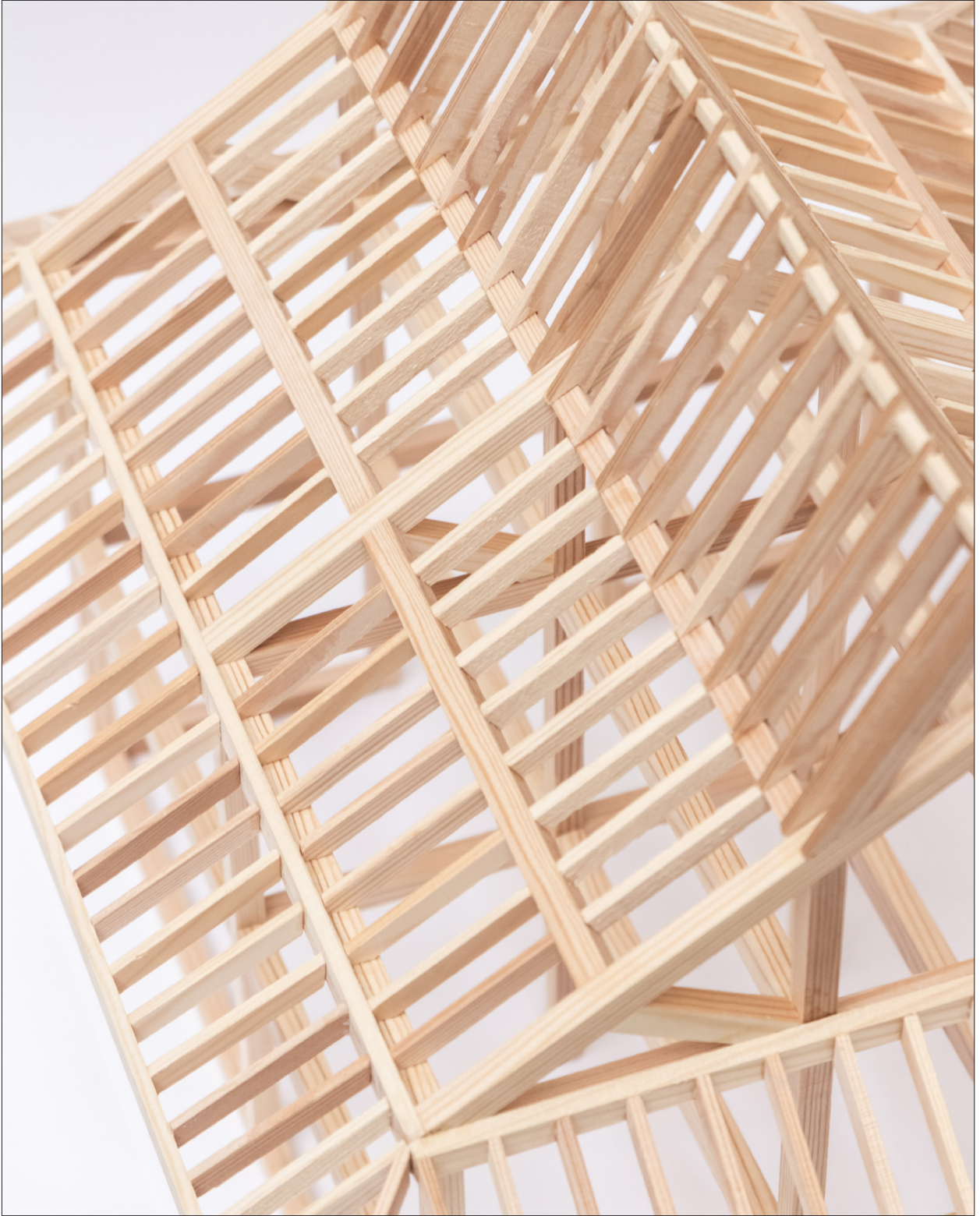
Detail of eaves and roof framing.
