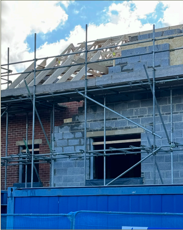
Fig. 2 Concrete masonry unit (CMU) and stick frame construction in Saffron Walden.
