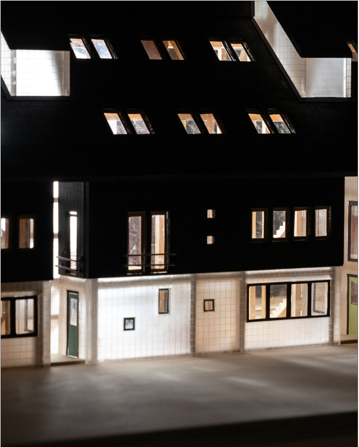
Glass blocks are used throughout the longhouse and bring light into the main stairwells while providing privacy.
