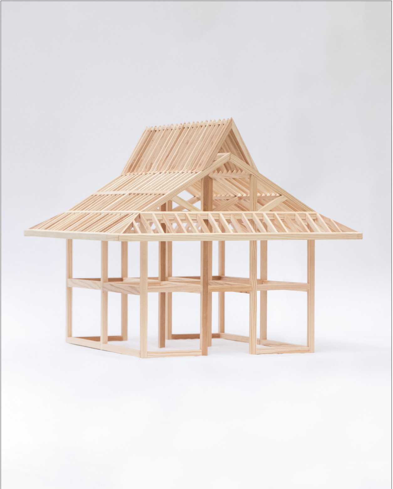
Framing model at 1:20 showing eaves.
