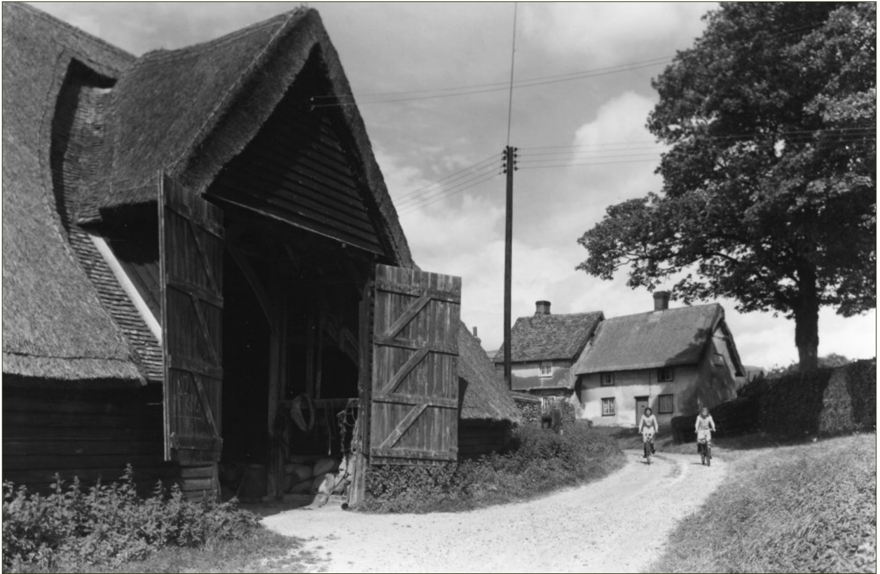
Fig. 1 15th century timber-framed barn with thatched roof, wattle and daub infill, and wood weatherboarding in Wendens Ambo, Essex. Via RIBAPix, reference RIBA42020.
