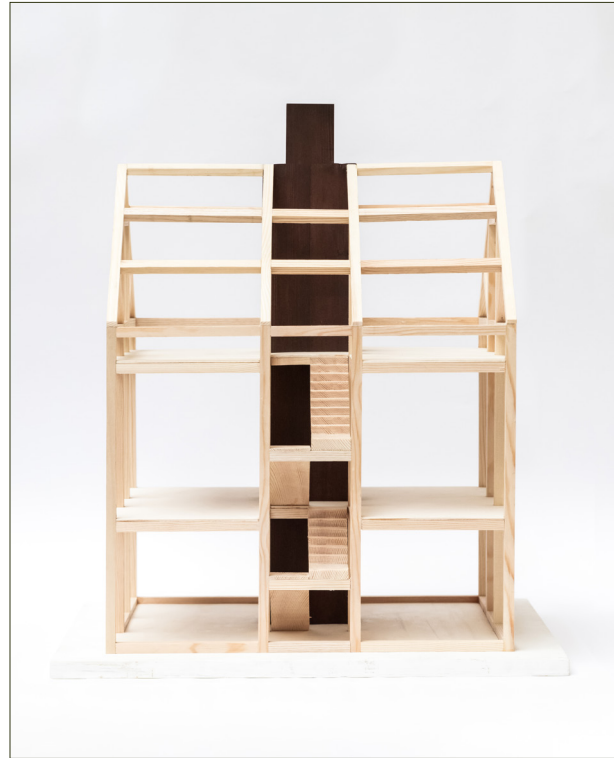
Fig. 3 1:50 Model of the 500-Year House. The Masonry stack (brown) concentrates all the electrical and plumbing, and provides easy access to wires and pipes.
