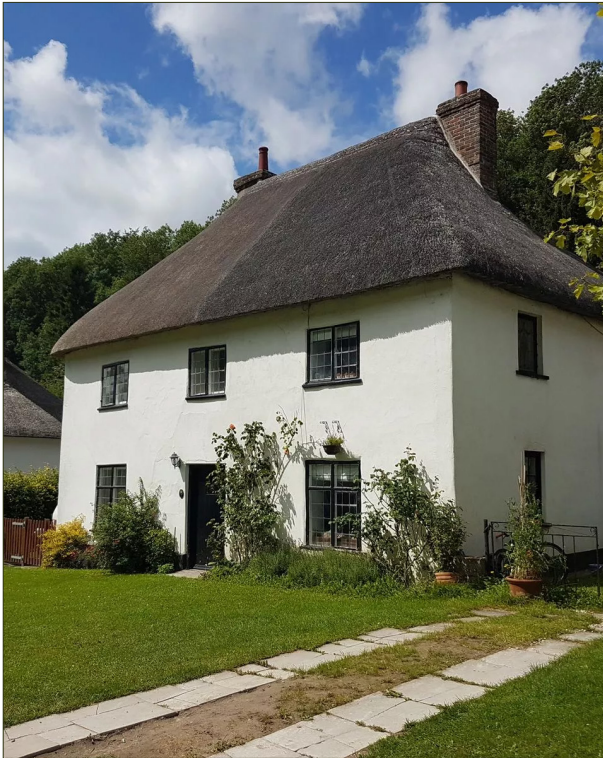
Fig. 1 Thatched roof and cob wall in Milton Abbas, Dorset. © Blackmore Vale Magazine/Reach
