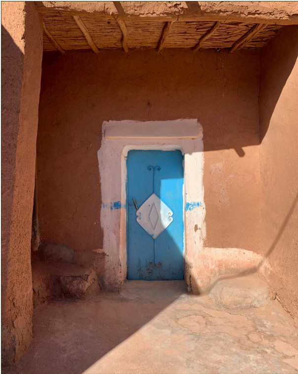
Fig. 2 Adobe building in Morocco. Many Moroccans still build their homes with adobe due to its thermal mass. This trip also inspired the use of lime-based Tadelakt plaster in this thesis.
