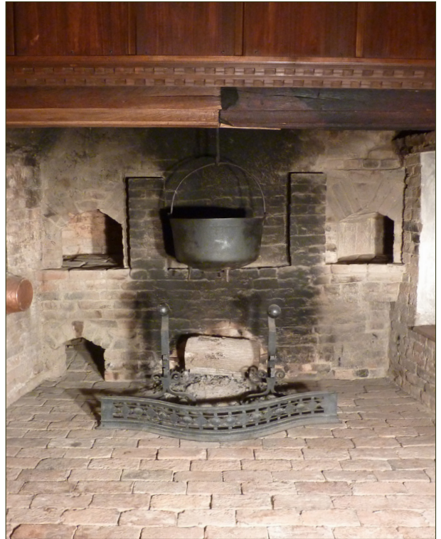
Fig. 17 Inglenook fireplace at Lummus House in brick and timber. Summer fires can be lit in the nooks on the rear wall. © A. Boynton via Flickr.
