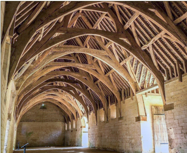
Fig. 20 Cruck trusses at Avon Tithe Barn, ca. 14th century.
