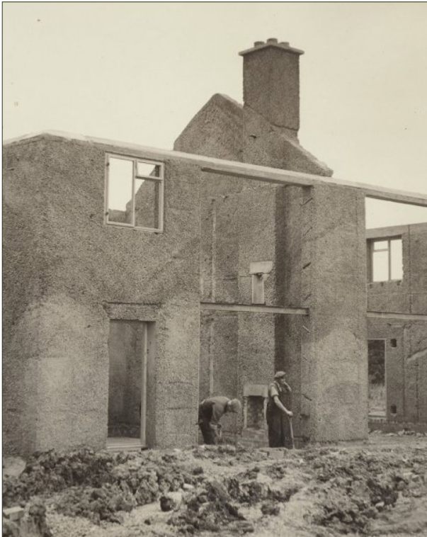
Fig. 11 Concrete and steel prefab housing in Hillingdon, 1949. © Hulton Archive/Getty Images via Science Museum Group
